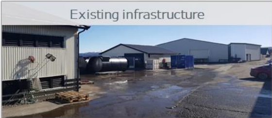
Capacity for 4.5k tonnes
